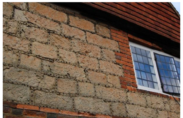
Figure 11: Photograph of the architectural technique 'galletting'
