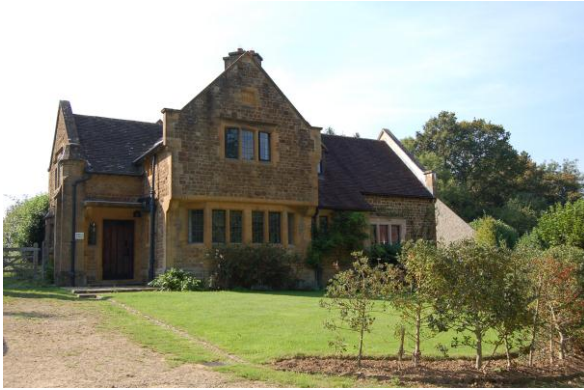
Figure 16: Witley Lodge, Churchfields
